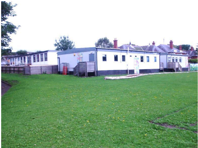
Ysgol Pen Barras mobile classrooms
